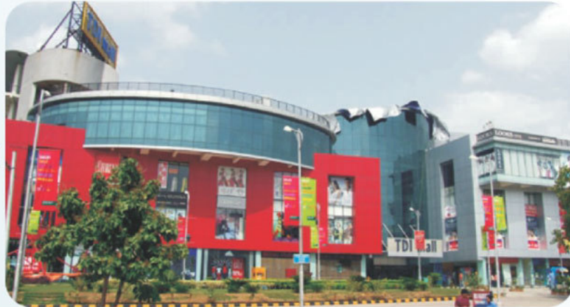
Commercial Project For TDI Group "TDI MALL" Area : 5.50 Lakh Sq.ft. (Approx) ◀ at Rajouri Garden, New Delhi
