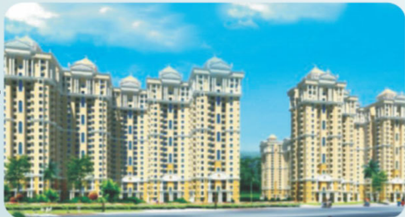
Residential Project For Nimbus Group "The Hyde Park" Area : 6 Lakh Sq.ft. (Approx) at Noida
