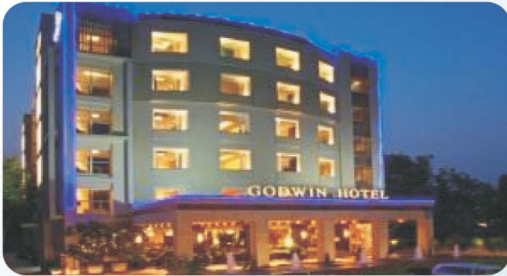
Commercial Project For Godwin Group "Godwin Hotel" Area : 2.50 Lakh Sq.ft. (Approx) at Haridwar
