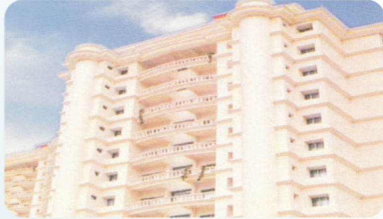
Residential Project For Shipra Group "Sun Tower" Area : 6 Lakh Sq.ft. (Approx) ◀ at Indirapuram
