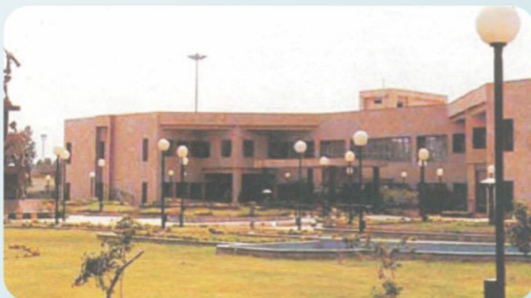
Institutional Project For NTPC “Administrative Building” Area : 2.50 Lakh Sq.ft. (Approx) (1000 Nos. Capacity Auditorium) at Dadri, Ghaziabad
