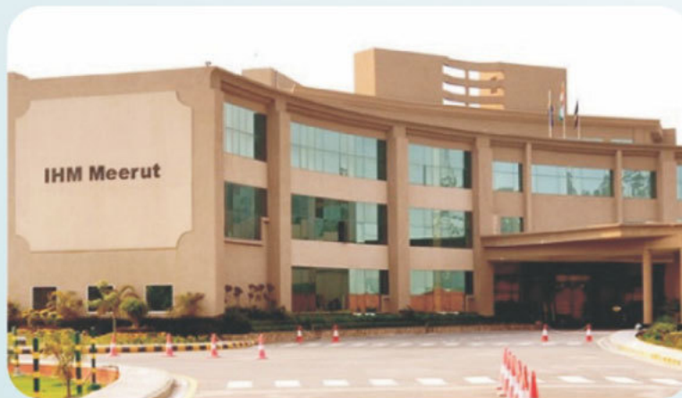
Institutional Project For IHM Group "Institutional Building" Area : 4.50 Lakh Sq.ft. (Approx) ▶ at Meerut
