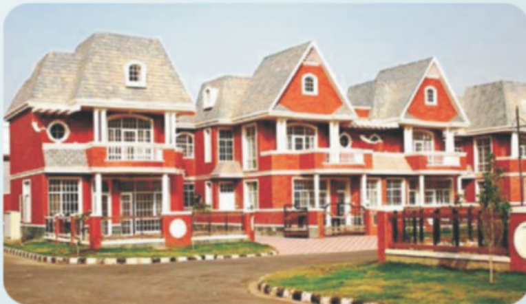
Residential Project For Eldeco Group "Eldeco Mensionz" Area : 2.50 Lakh Sq.ft. (Approx) at Gurgaon
