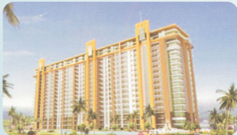
Residential Project For Pal Group "Pal Greens" Area : 6 Lakh Sq.ft. (Approx) ◀ at Faridabad
