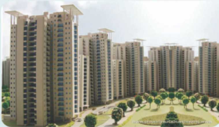
Residential Project For Jaypee Group "Aman Towers" Area : 16 Lakh Sq.ft. (Approx) at Noida
