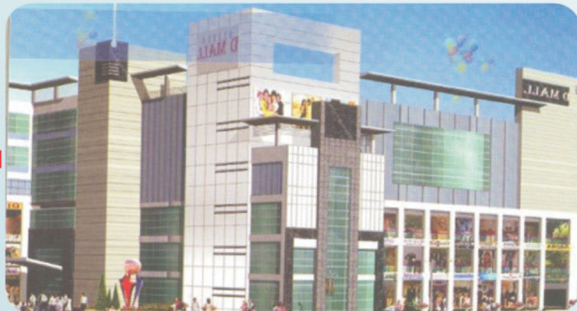
Commercial Project For Deep Ganga Group "D.G Mall" ◀ Area : 3 Lakh Sq.ft. (Approx) at Haridwar
