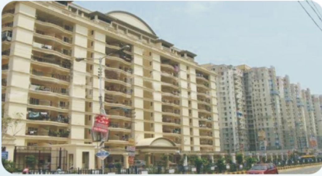
Residential cum Commercial Project For Shipra Group “Shipra Krishna” Area : 9 Lakh Sq.ft. (Approx) at Indirapuram, Ghaziabad
