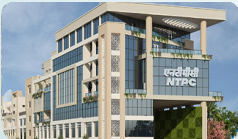
Construction of ER-II Hq Office Building & Residential Complex For "NTPC" Area: 92500 Sq.ft. (Approx) at Bhubaneswar, Odisha
