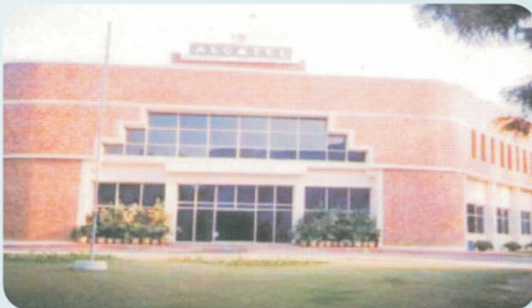
Commercial Project For Alcatel Group "Alcatel Network System Industrial Building" Area : 3 Lakh Sq.ft. (Approx) at Gurgaon
