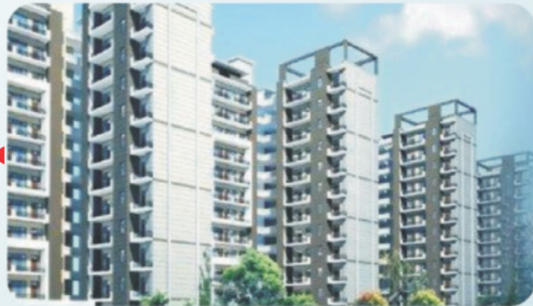
Residential Project For Landmark Group "Kunjeans Heights" ▶ Area : 6 Lakh Sq.ft. (Approx) at Faridabad
