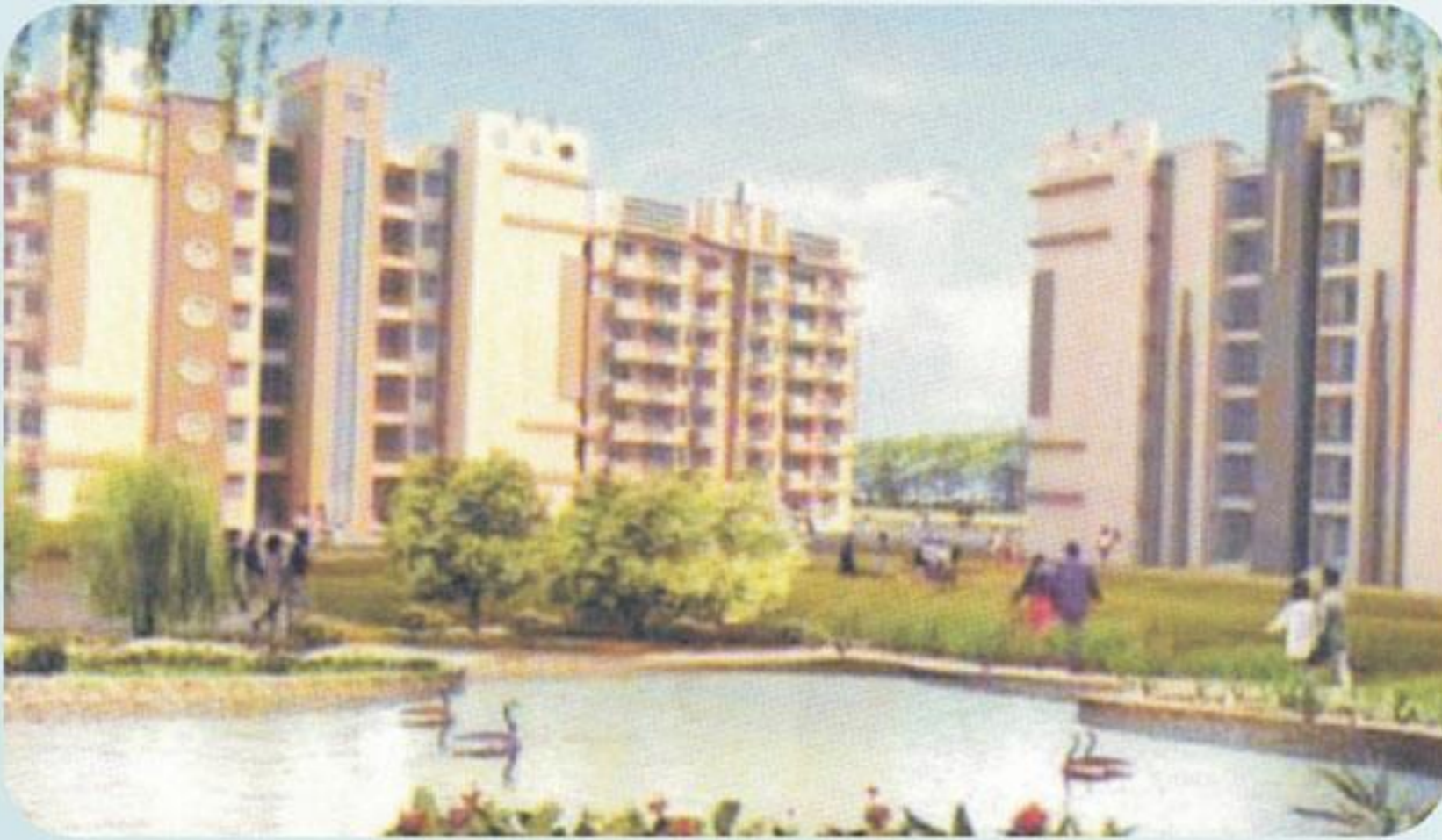
Residential Project For Horizon & Ascent Group "Kings Garden" Area : 2.70 Lakh Sq.ft. (Approx) at Jalandhar
