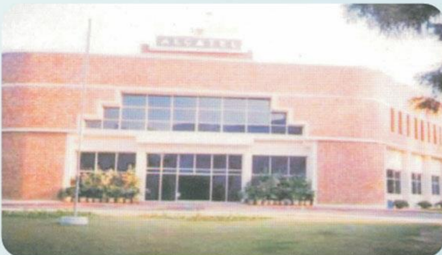
Commercial Project For Alcatel Group "Alcatel Network System Industrial Building" Area : 3 Lakh Sq.ft. (Approx) at Gurgaon
