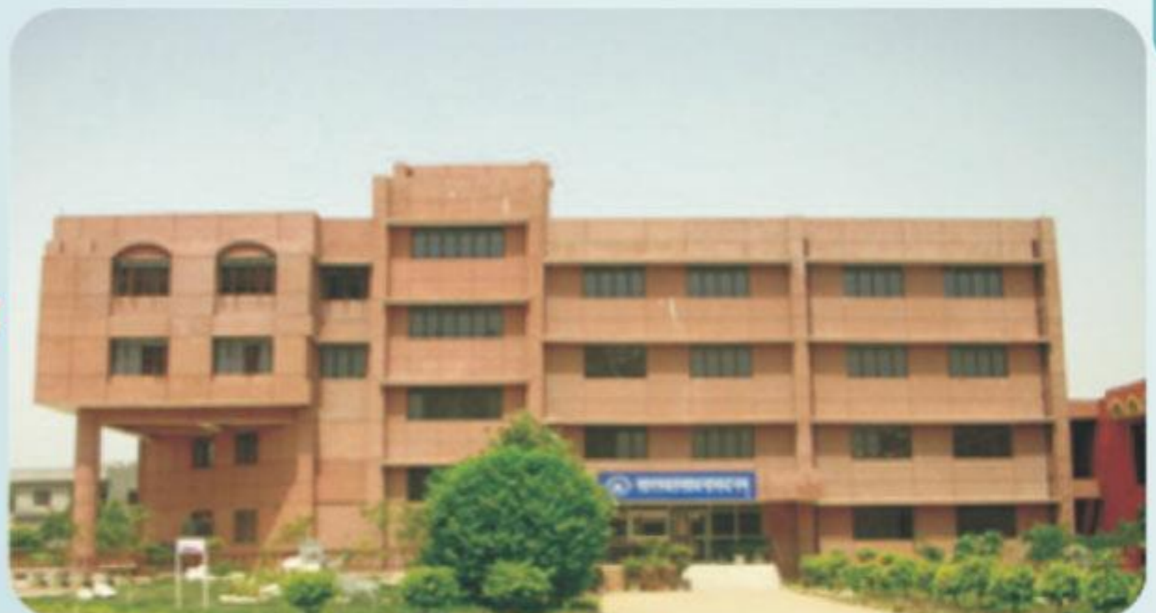
Institutional Project For L.B.S.V “Administrative Block Building” Area : 2 Lakh Sq.ft. (Approx) at Katwaria Sarai, Delhi
