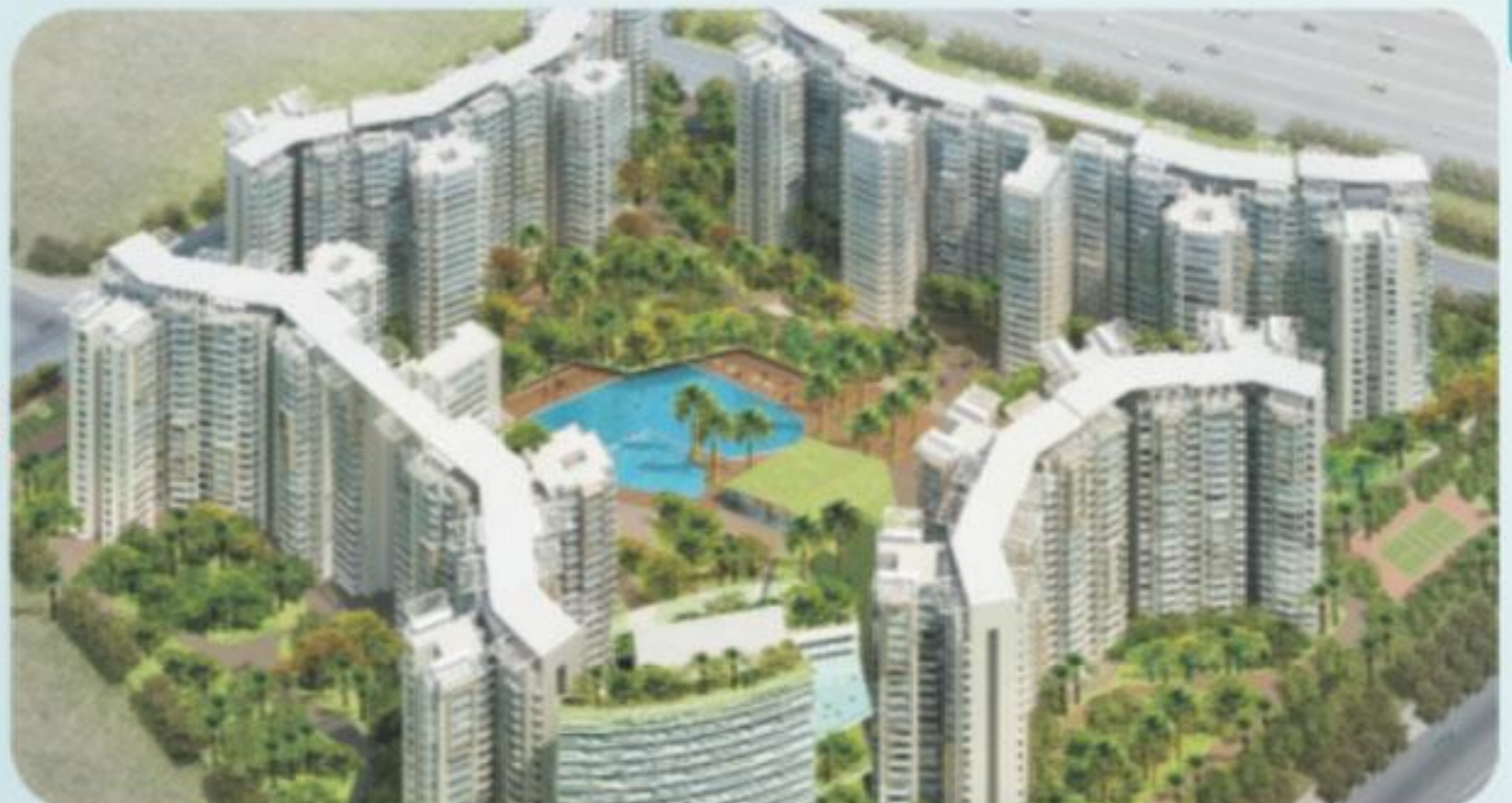
Residential Project For Pan Group "Pan Oasis" Area : 6 Lakh Sq.ft. (Approx) at Noida
