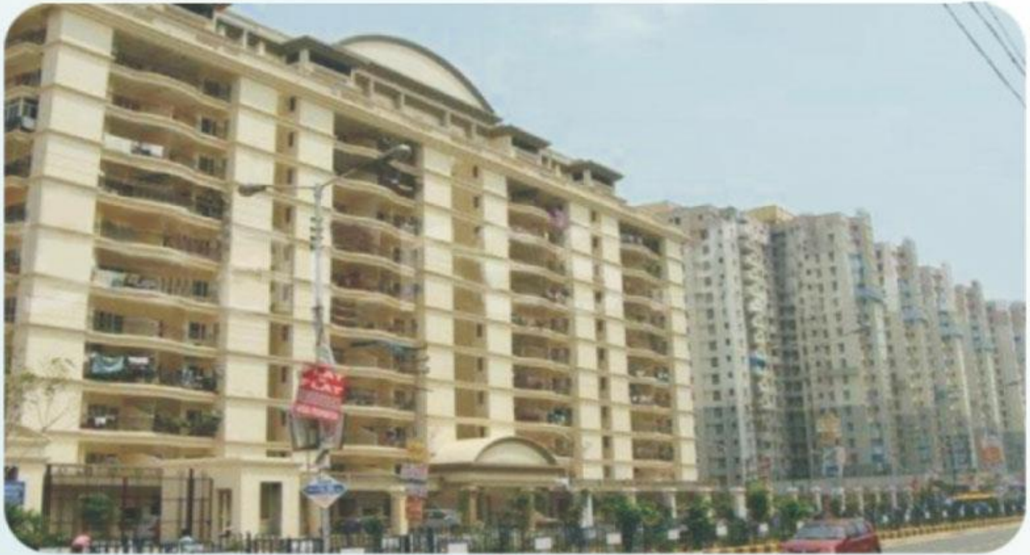
Residential cum Commercial Project For Shipra Group "Shipra Krishna" Area : 9 Lakh Sq.ft. (Approx) at Indirapuram, Ghaziabad
