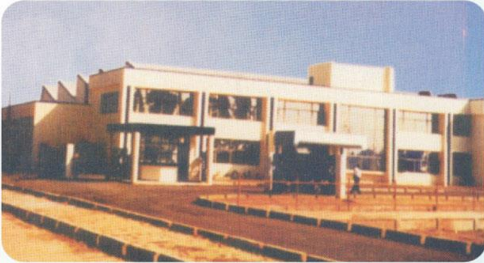
Commerical Project For "Krishna Boysen Exhaust Ltd." ▶ Area : 1.5 Lakh Sq.ft. (Approx) at Greater Noida
