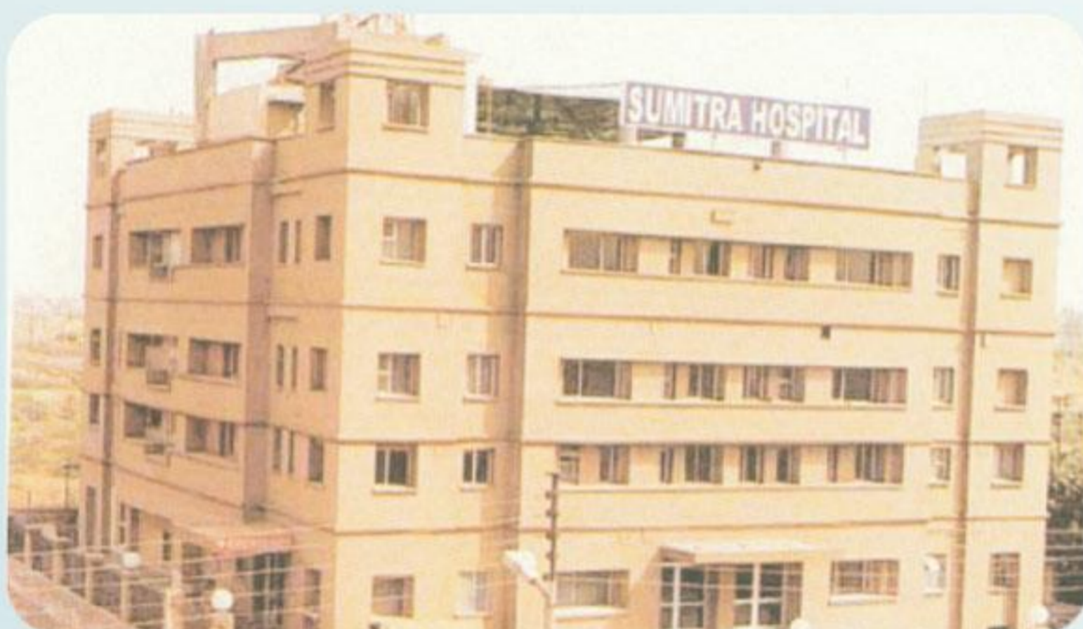
Commercial Project For "Sumitra Hospital" Area : 50 Thousand Sq.ft. (Approx) ▶ at Noida
