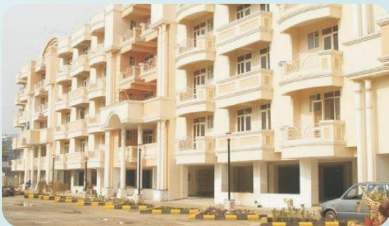
Residential Project For Hansmukhi & Ascent Group "Race Course Valley" Area : 4.20 Lakh Sq.ft. (Approx) at Dehradun
