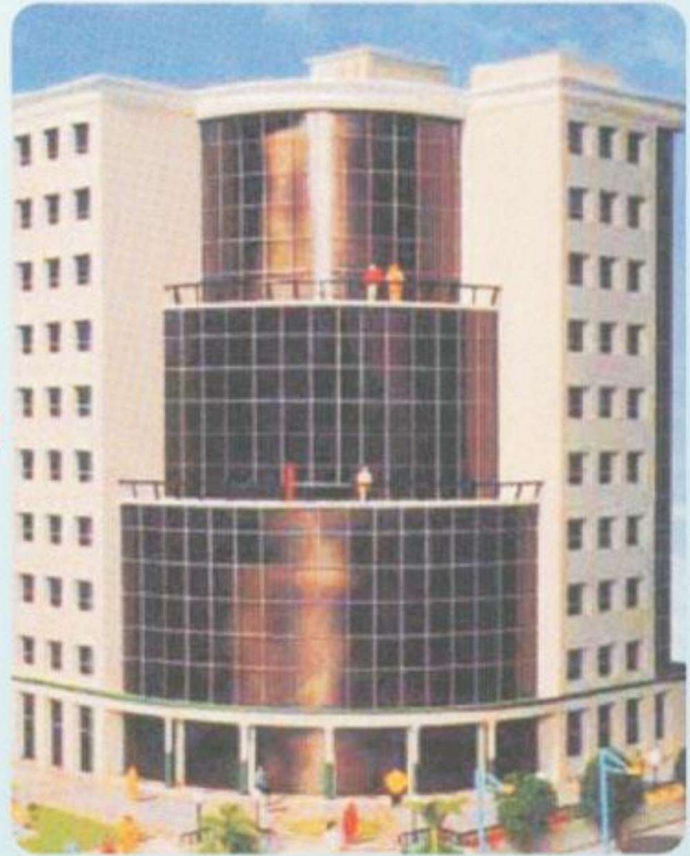
Commercial Project For Niti Shree Group "Shopping cum Office Complex Tradex Tower-II" (3 Tower) Area : 3 Lakh Sq.ft. (Approx) at Greater Noida
