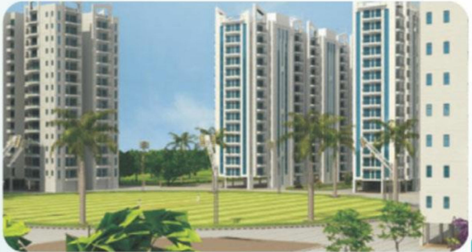
Residential Project For VVIP Group "VVIP Addresses" Area : 8 Lakh Sq.ft. (Approx) at Raj Nagar Extn, Ghaziabad
