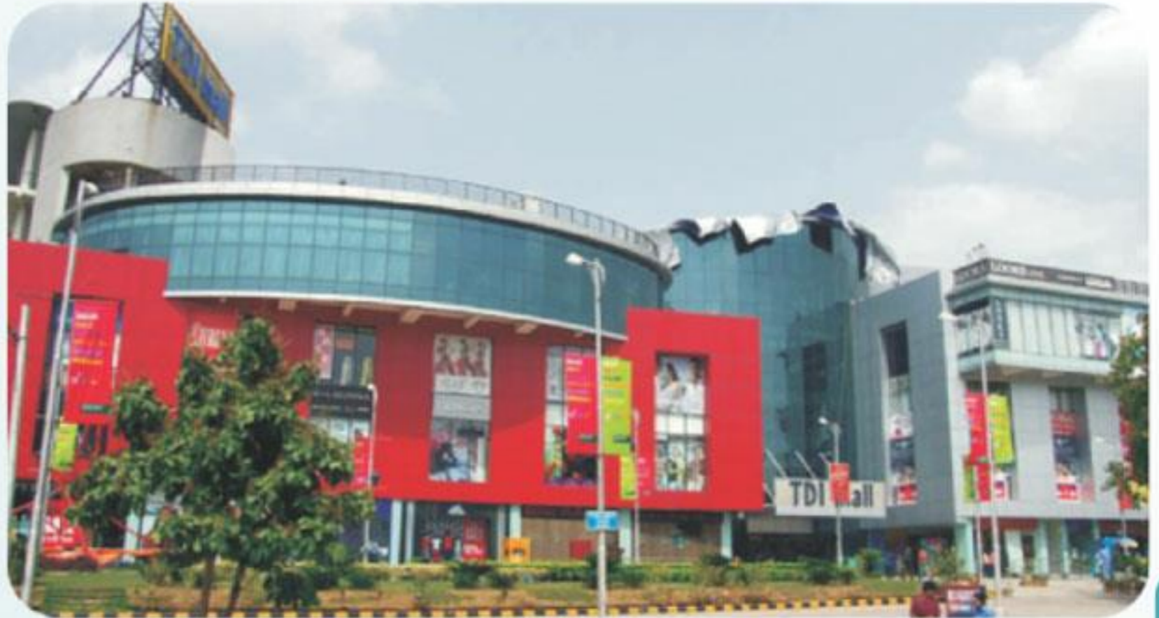
Commercial Project For TDI Group "TDI MALL" Area : 5.50 Lakh Sq.ft. (Approx) ◀ at Rajouri Garden, New Delhi
