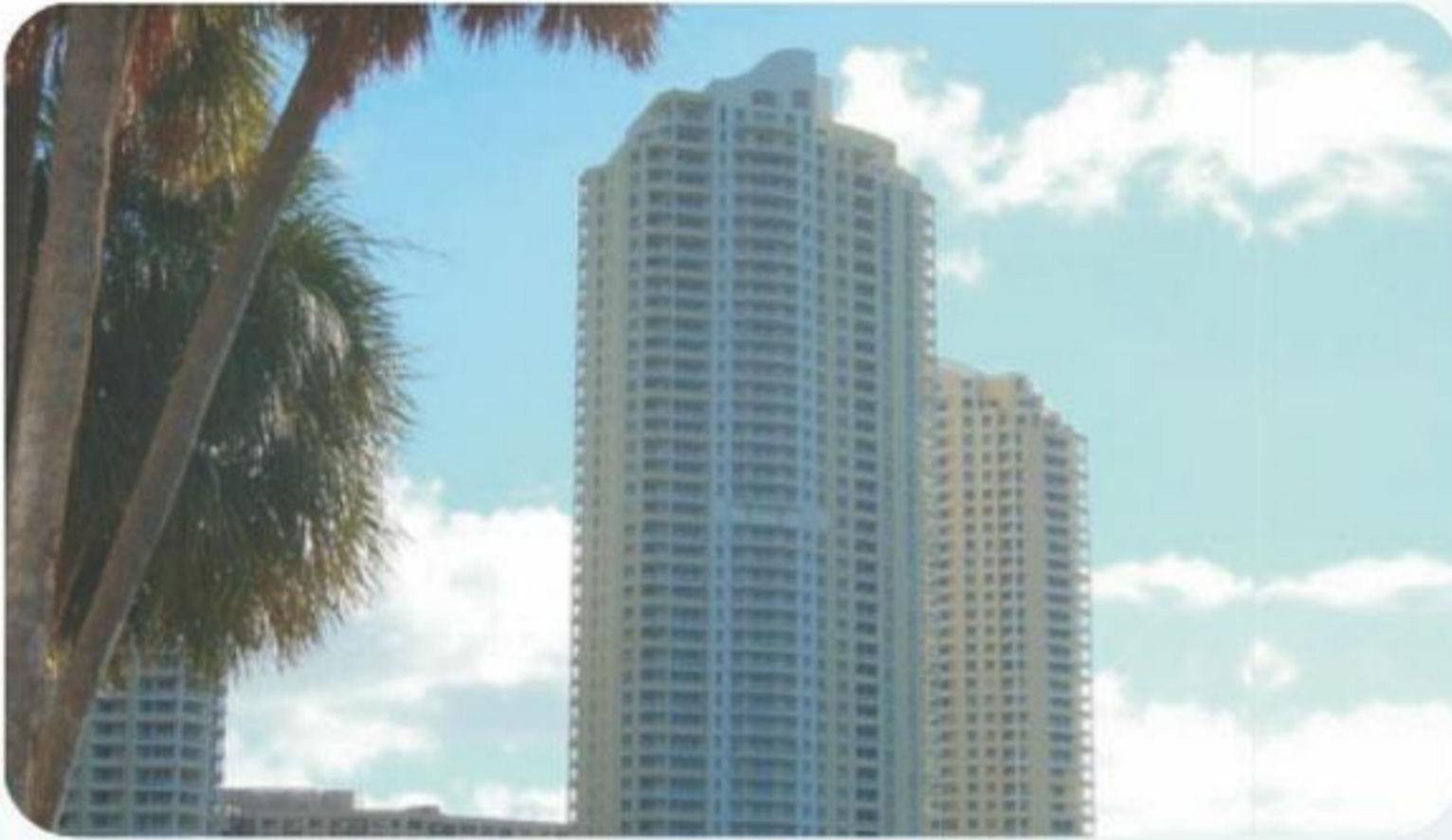
Residential Project For M2K Group "County Heights" Area : 8 Lakh Sq.ft. (Approx) at Daruhara, Sec-5, Gurgaon
