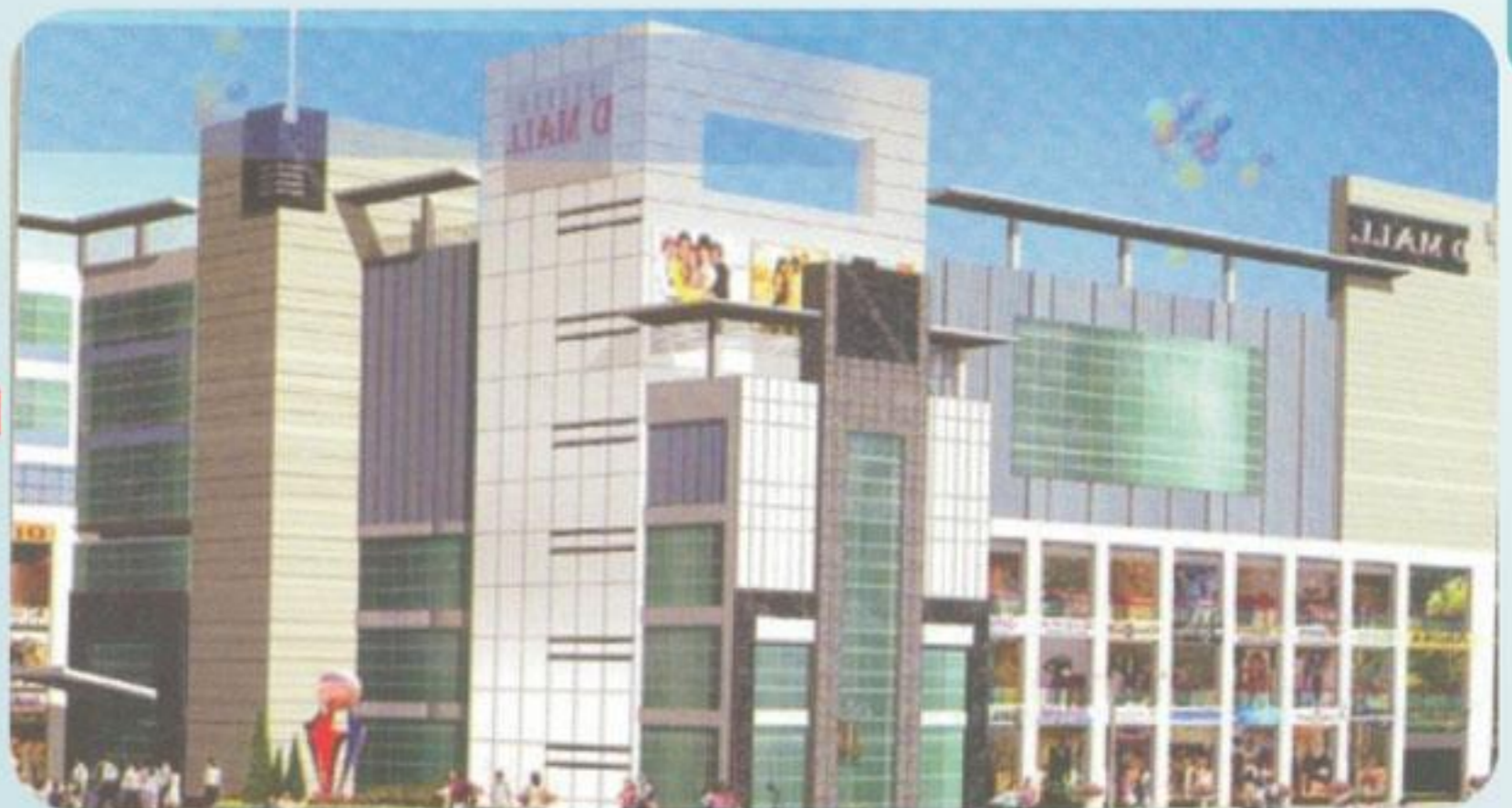
Commercial Project For Deep Ganga Group "D.G Mall" ◀ Area : 3 Lakh Sq.ft. (Approx) at Haridwar
