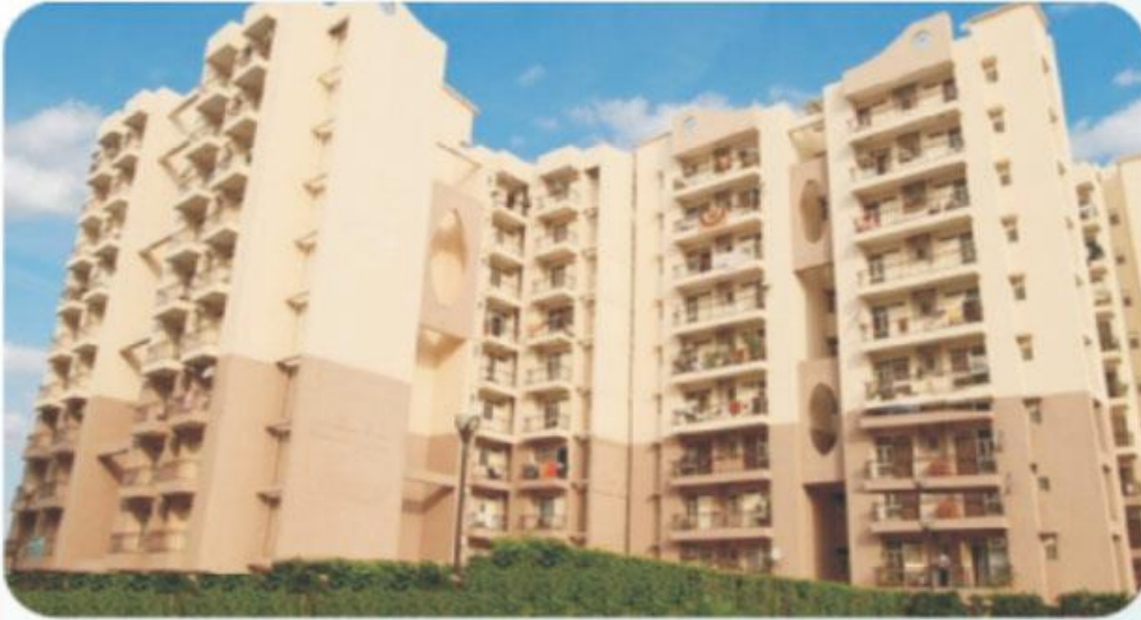
Residential Project For Landcraft Group "River Heights" Area : 3 Lakh Sq.ft. (Approx) at Raj Nagar Extn, Ghaziabad
