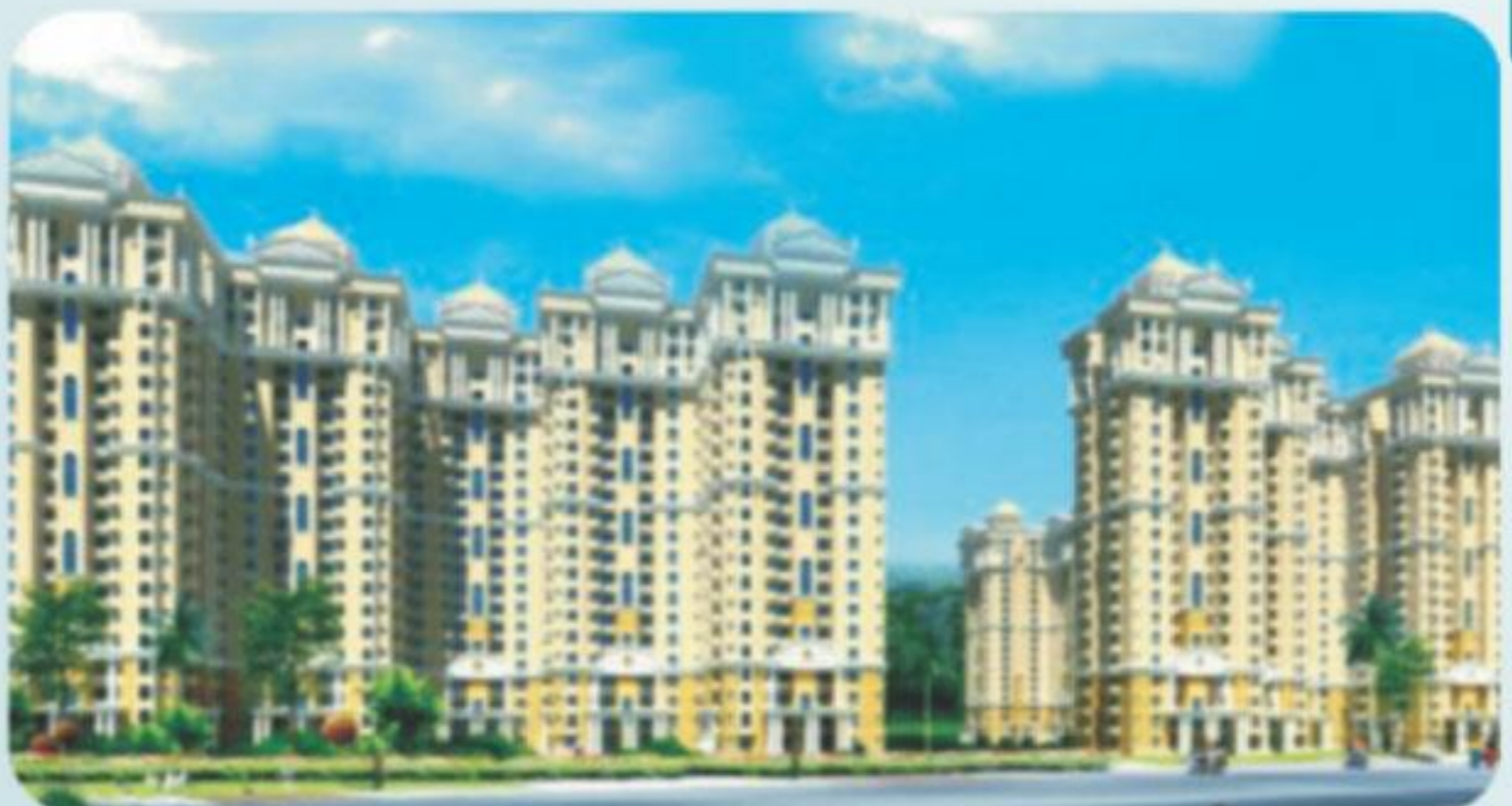
Residential Project For Nimbus Group "The Hyde Park" Area : 6 Lakh Sq.ft. (Approx) at Noida
