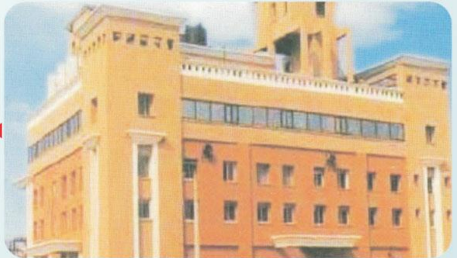
Commercial Project For "Prakash Hospital" Area : 1 Lakh Sq.ft. (Approx) ◀ at Noida
